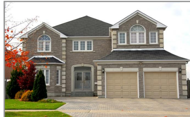
Combined heat and power (CHP)
